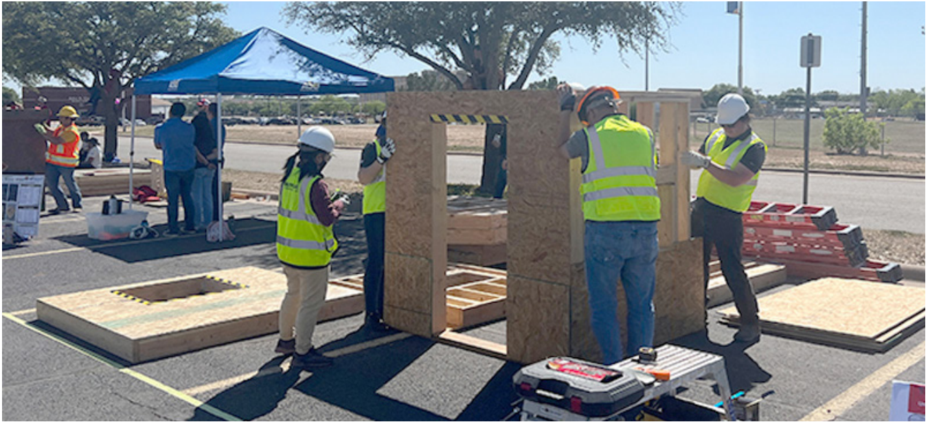
Student-led teams have 90 minutes to erect attractive, durable, engineered wood structures.
